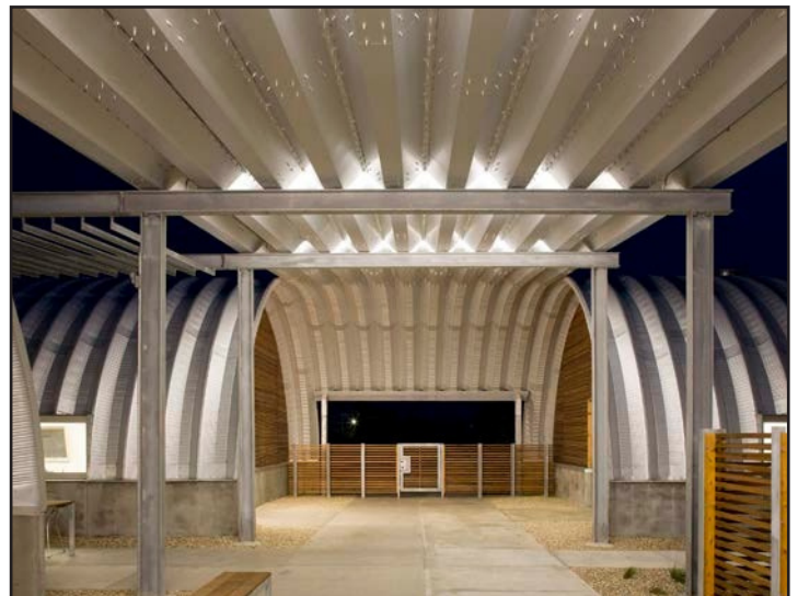
Owner: Tangipahoa Consolidated Gravity & Drainage District No. 1 Architect: Holly and Smith Architects, APAC General Contractor: Ragusa Construction, LLC Photographer: Marc Lamkin Photography
